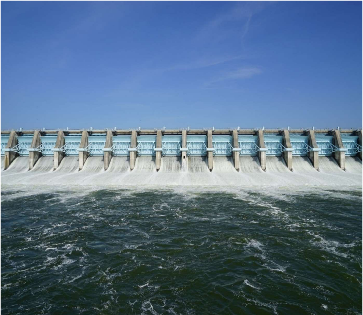
Spillway at Richland Chambers
