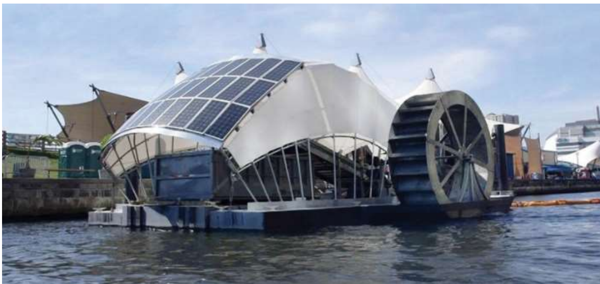
Pictured above is a water wheel structure designed to pull trash out of the waterways.
