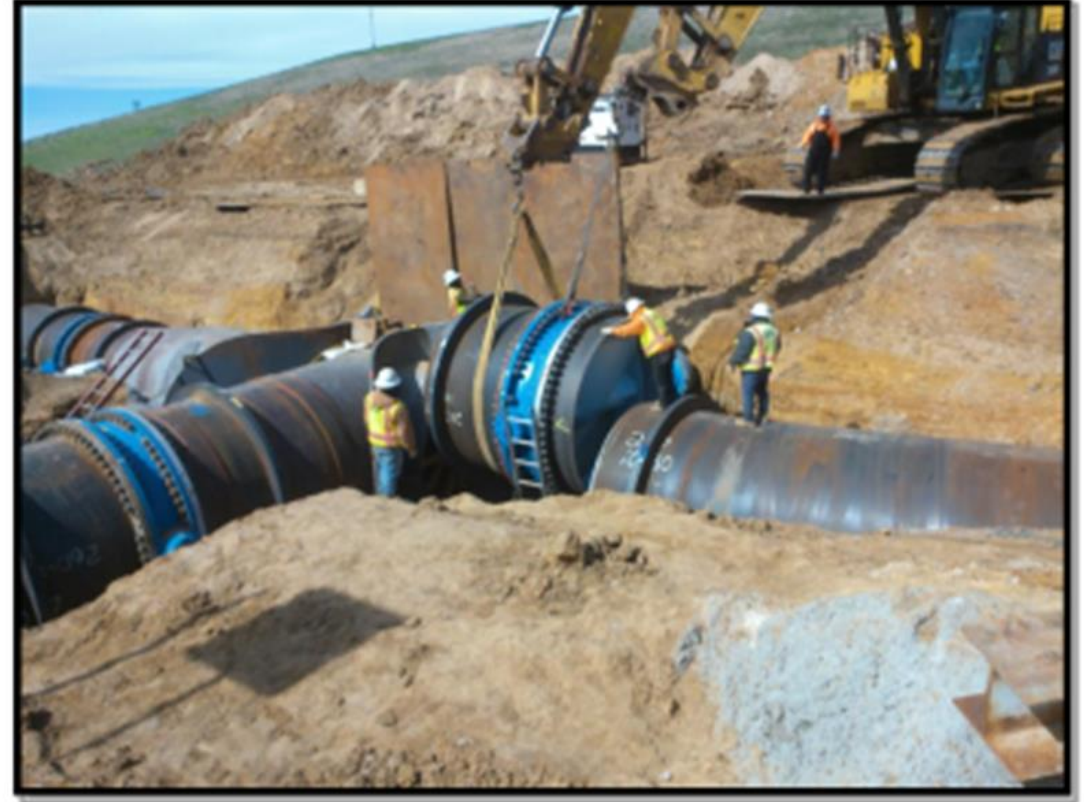
BAR laying valve T466
