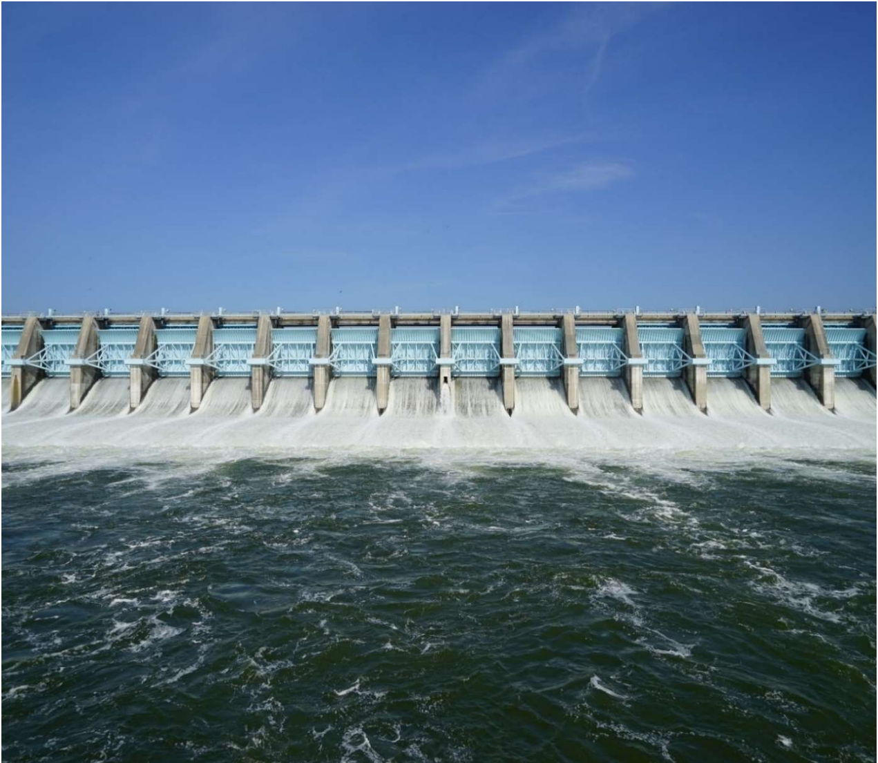
Spillway at Richland Chambers
