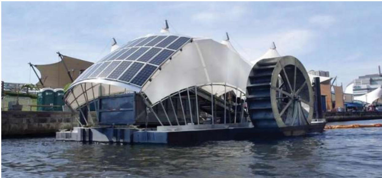
Pictured above is a water wheel structure designed to pull trash out of the waterways.
