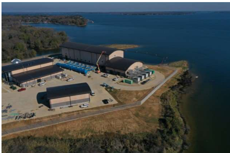
The Joint Cedar Creek (JCC1) pump station came online in fiscal year 2023, increasing pumping capacity and the need for additional chemicals.
