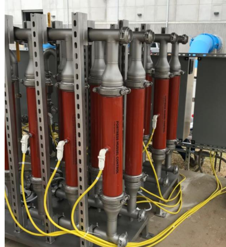
$2.5M copper ion addition for zebra mussel control at Benbrook Lake PS
