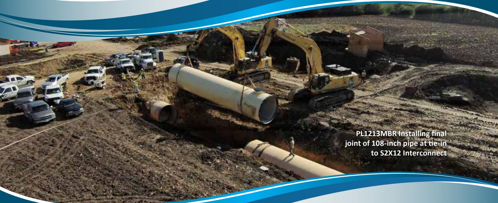
PL1213MBR Installing final joint of 108-inch pipe at tie-in to S2X12 Interconnect
